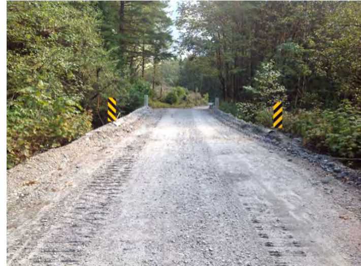
Approach from Right Bank when facing downstream
