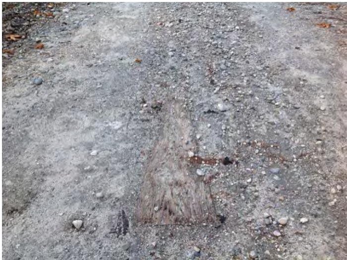
exposed stringer at left approach
