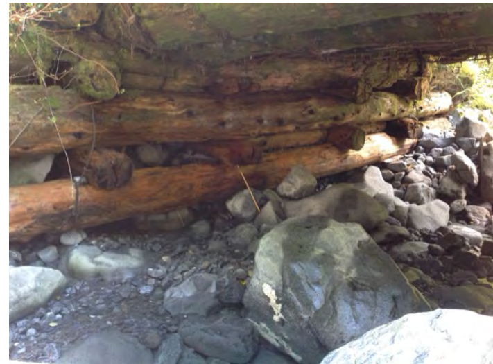
Left Bank Abutment when facing downstream
