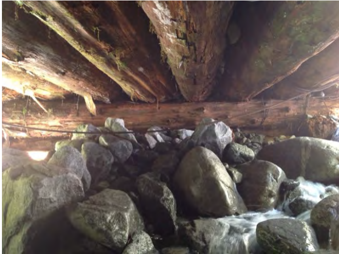
Right Bank Abutment when facing downstream
