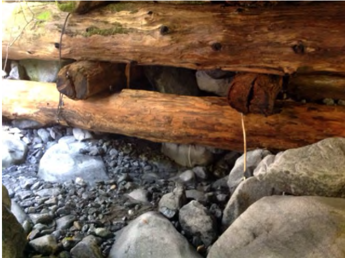
Left Bank Abutment when facing downstream
