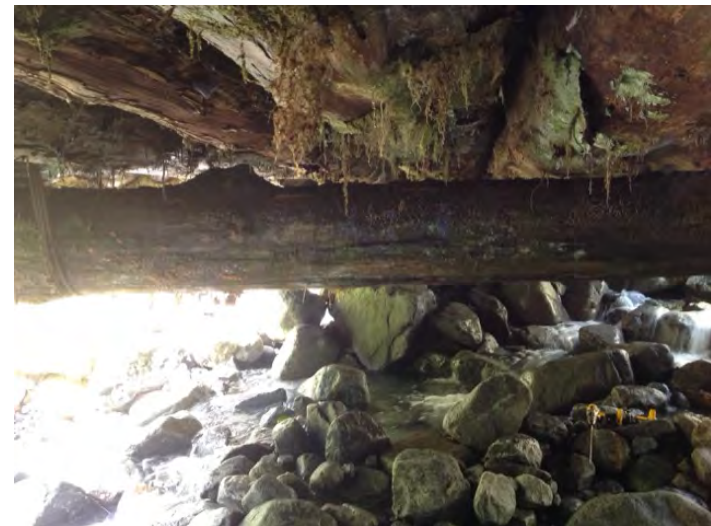
needle beam - not functional
